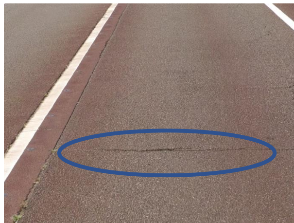
Figure 3 Transverse Cracks
