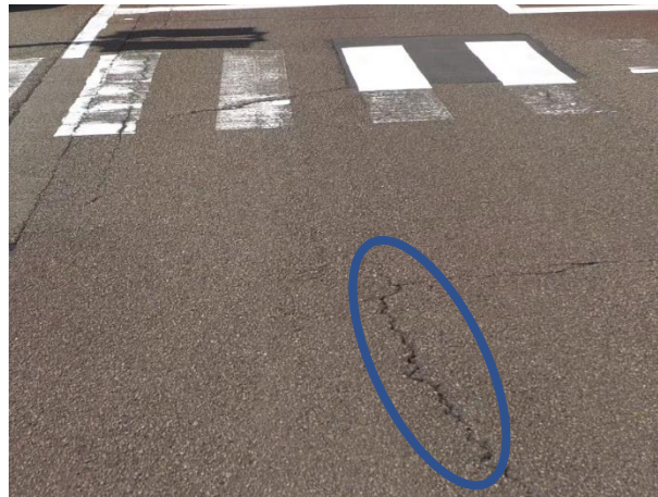
Figure 2 Longitudinal Cracks
