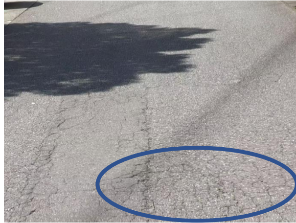
Figure 1 Alligator Cracks
